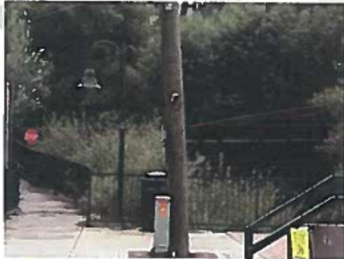
Figure 14. Pedestrian Lighting in Morrison
